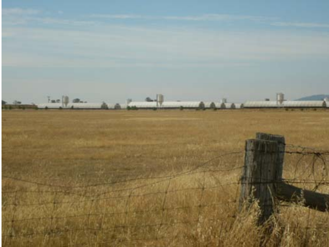
Part of the QAF multisite system at Gre Gre Victoria
