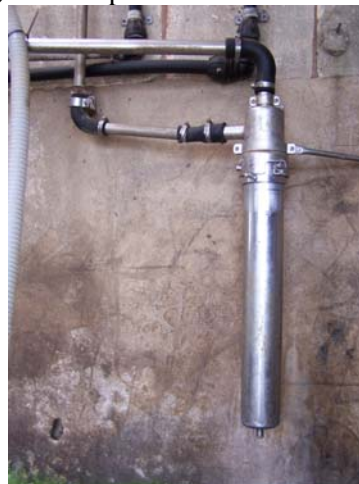
c) Screw open filter
