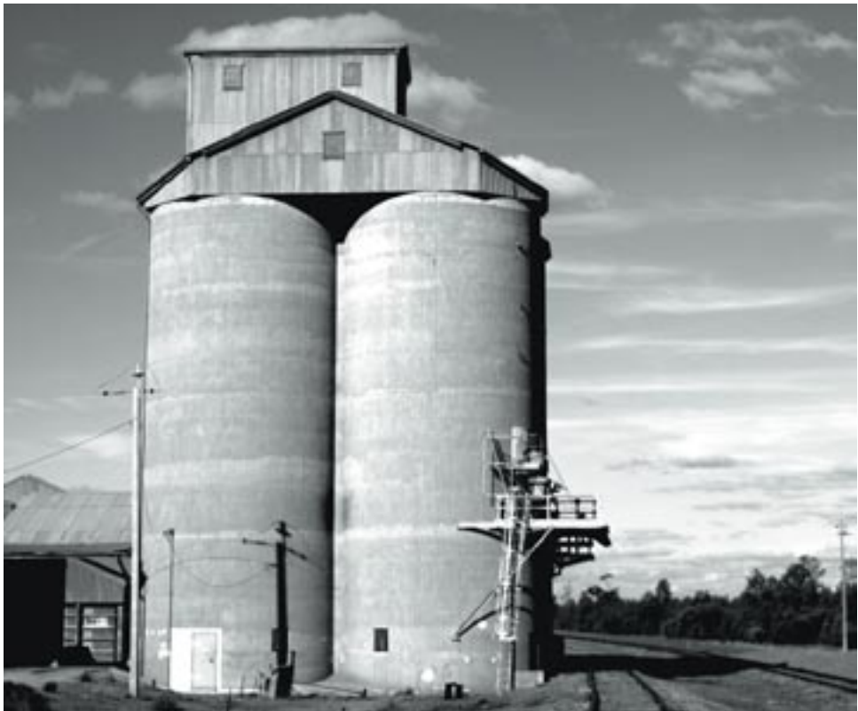
Silos near Griffith, NSW
