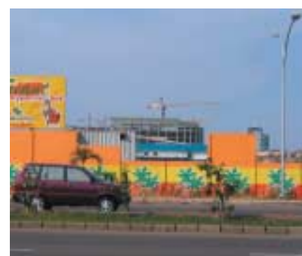
Image 3.13 Giant hypermarket under construction, Kelapa Gading, Jakarta
